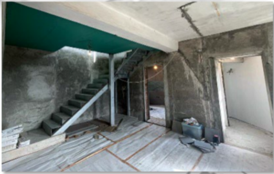
During reconstruction (Ground Floor)
