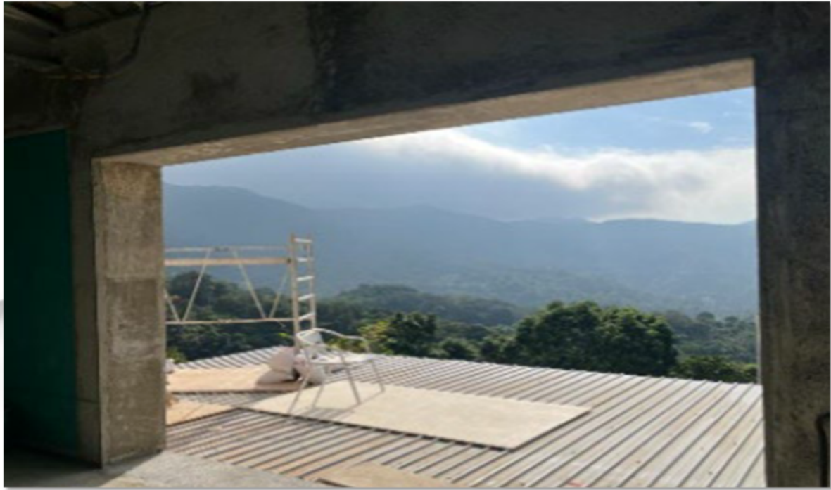
During reconstruction (First Floor)
